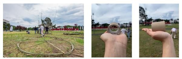
• On the 2nd day, we placed pruned wicker trees between the sections created and tied them with tie wires. We tried to strengthen the structure by tying the wicker branches more tightly.
