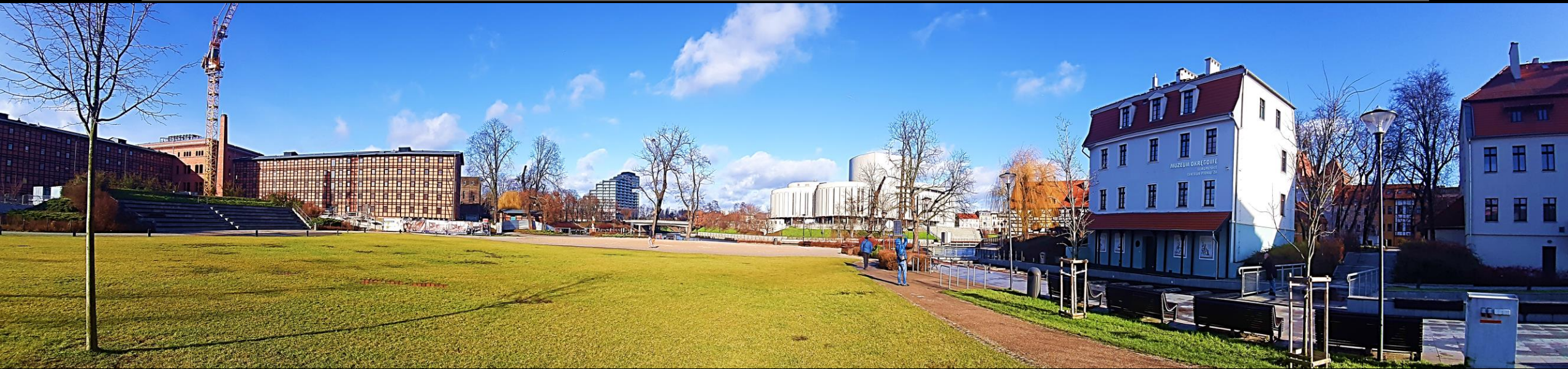
Figure 2. The revitalized space of the Mill Island from the east with the buildings of the District Museum L. Wyczółkowski, from the west side of Rother's Mill, from the north the Nordic Haven tower and Opera Nova. (source: author's photo)
