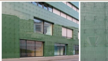
Figure 5. Institute for Hospital Pharmaceuticals, Basel, Switzerland (Herzog & de Meuron, 1998): A – the section of the building on the street side; B – elevation structure and graphical features. Photo: Maarten Helle.
