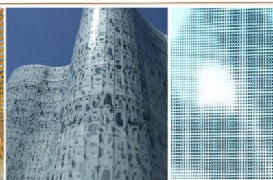
Figure 4. The University Library, Cottbus: A – building's façade; B – interference patterns from up close. Photos: by the author.
